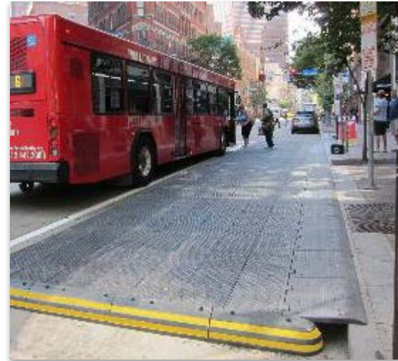
Bulb-outs to allow buses to board from the travel lane and provide more space for passengers to wait
