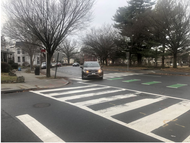
Exiting vehicle making a turn at a poor conflict angle with the bicycle lane and crosswalk
