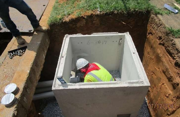
Structure tied into conduit
