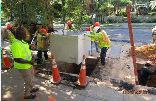
Structures lifted into excavated hole
