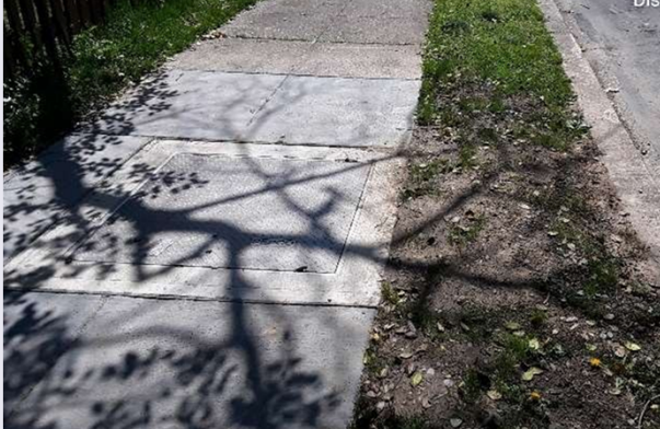
Final restoration tap hole
