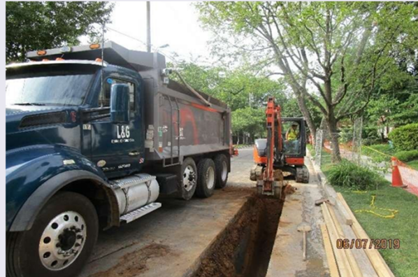
Trench is excavated
