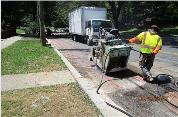
Marked & saw cut
