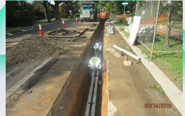
Conduit is laid
