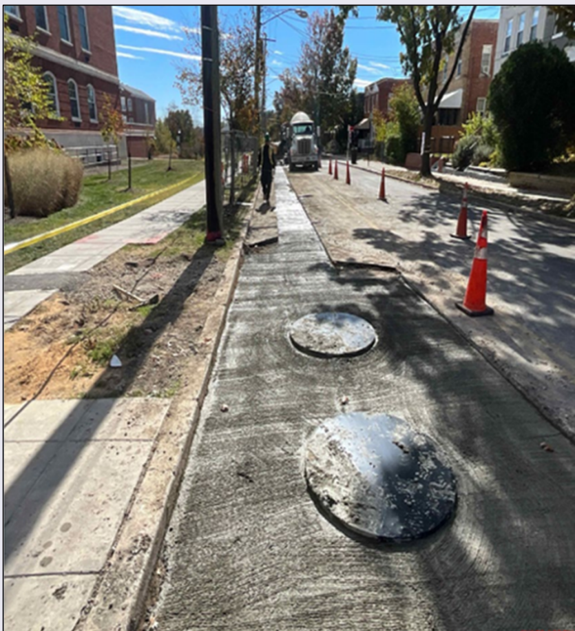
Final restoration of manhole
