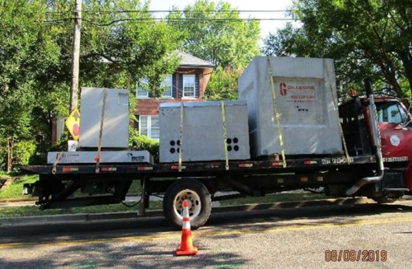
Tap hole, Transformer Enclosure, Manholes
