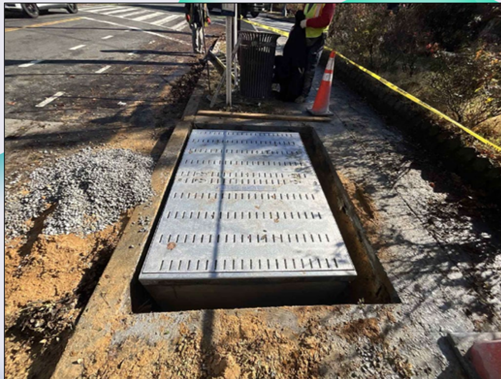
Final restoration of transformer enclosure
