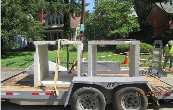
Structures delivered to site
