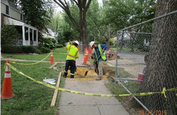
Structure is capped off & backfilled
