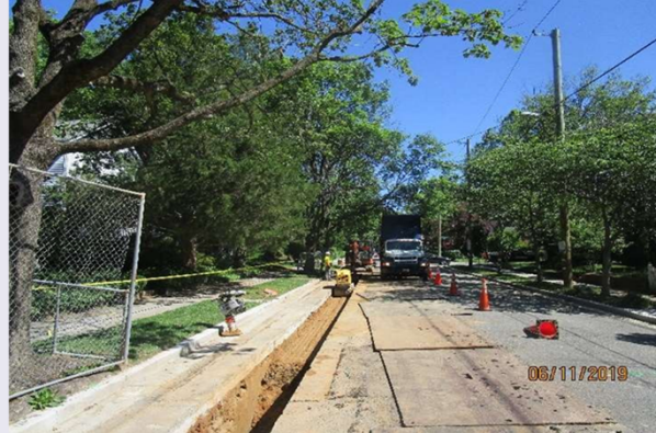
Trench is backfilled, then temporarily covered
