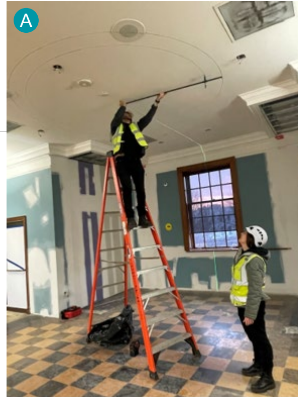
Ceiling preparation in the Children Story Time Space.
