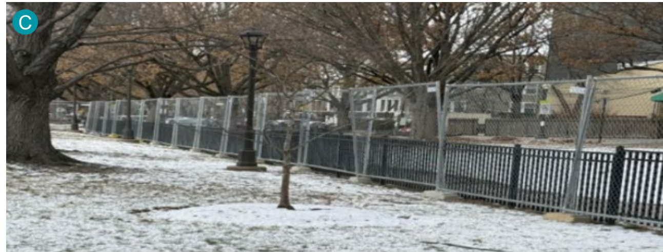
Construction fence along Iowa Ave. NW and Route 29
