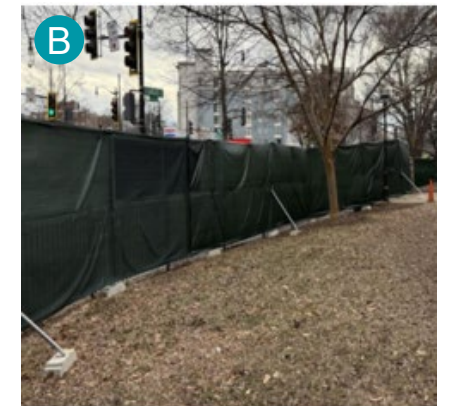
Construction fence along Upshur St. NW
