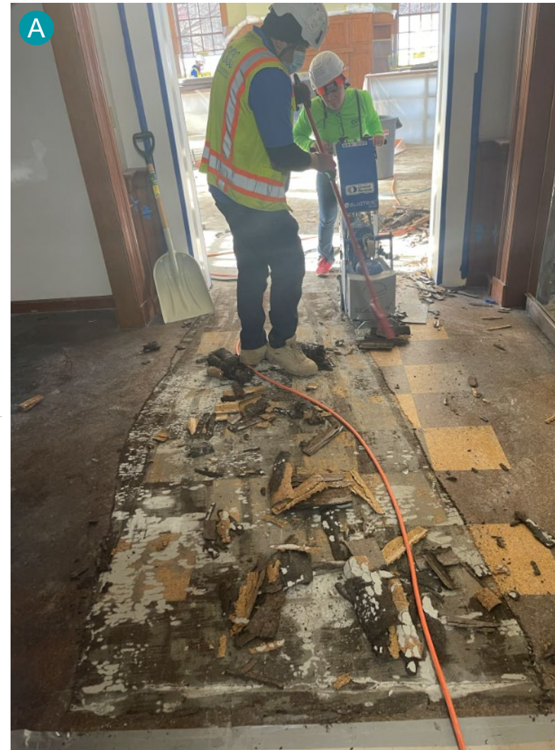
Old cork floor removal in progress by the West Stair.
