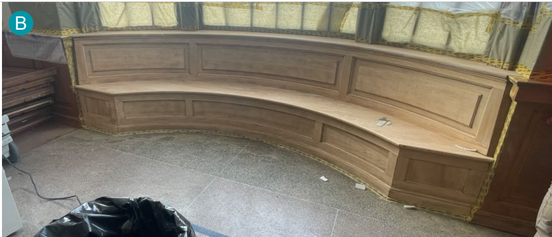
Existing bench in the new Seating Space sanded.
