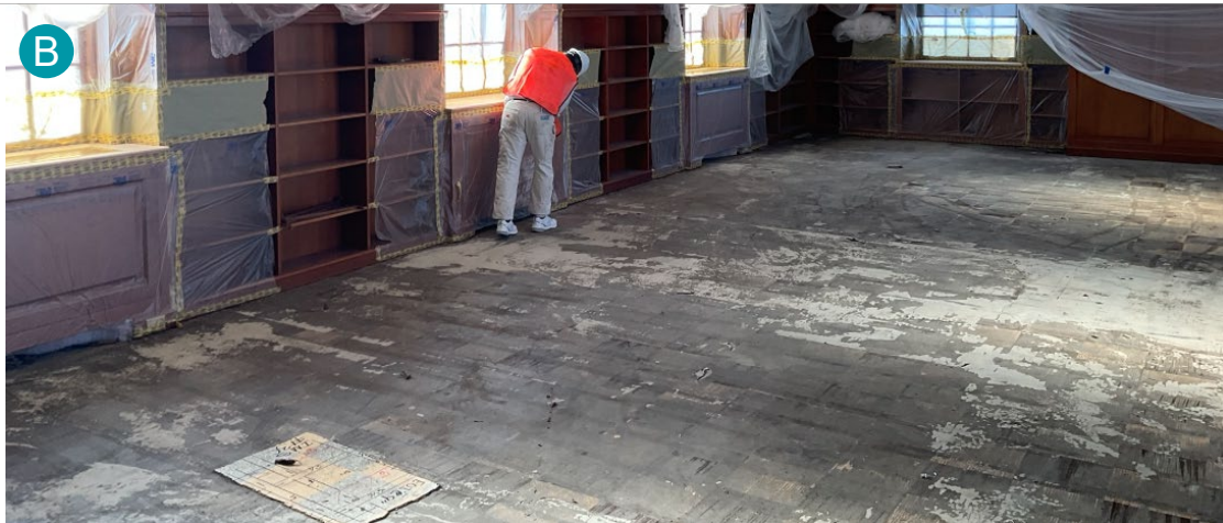
Old cork floor removal completed in the Adult Area.
