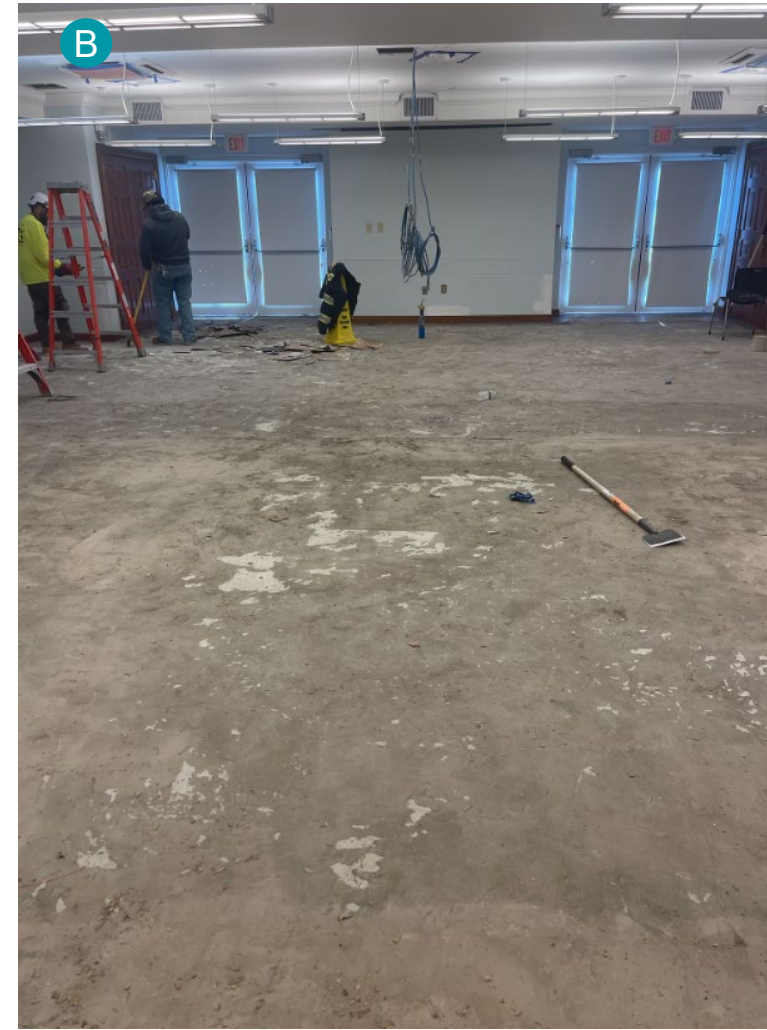
Floor removal in the Meeting Room.
