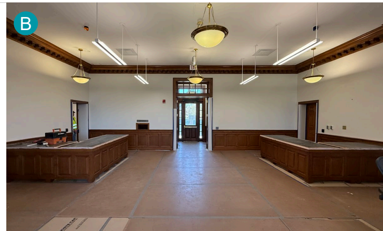
Refinishing the main service desk, cleaning the historic light fixtures, and installation of the new lights is complete. Refinishing the front door and painting of the walls is in progress.
