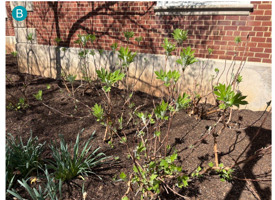
Exterior patch repair near the front entrance completed and planting restored.
