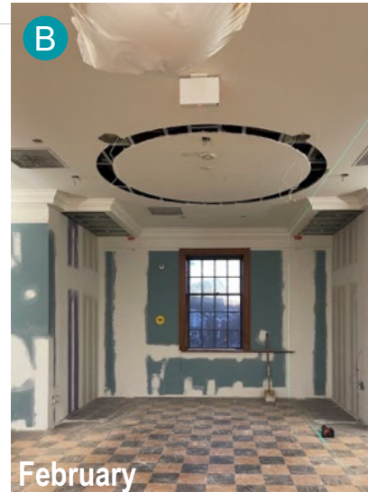
Installation of the hung acoustic balloon fixture and lighting is near completion. Reconfiguration of the crown molding and wall painting is complete.
