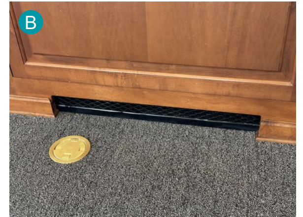
Installation of the floor boxes and new radiator grills complete.
