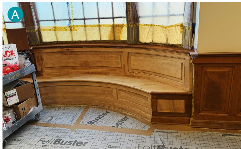
Progress in March: Refinishing the Reading Area wooden bench in progress.
